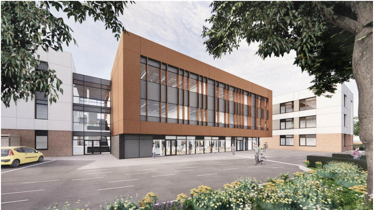
Figure 4: View from the new student and visitor entrance from Elm Park
